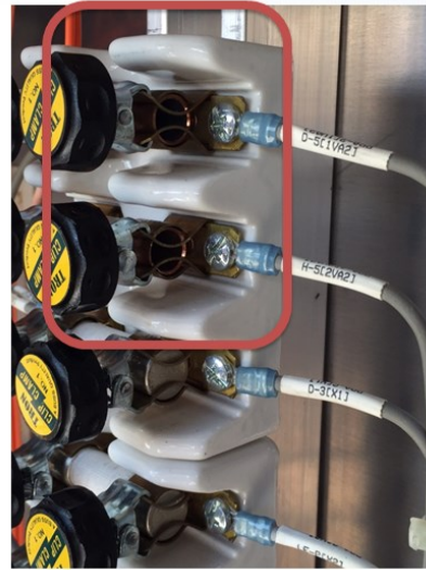
Figure 6 - Picture of Incorrect Shorting Slugs
