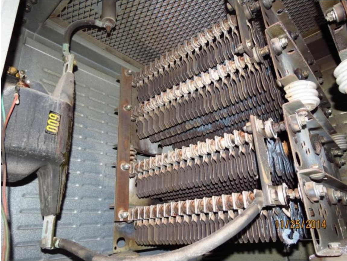
Figure 4. Damaged Common Neutral Resistor at S Street
