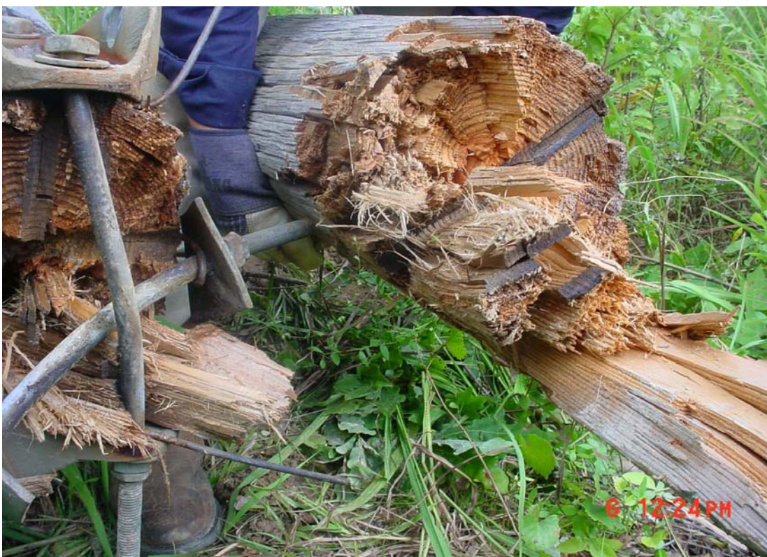
Figure 17. Broken Pole/Crossarm of Structure 566 - Source of Intermittent Fault
