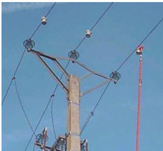
Fig 2. Overhead clip-on fault passage indicators.
