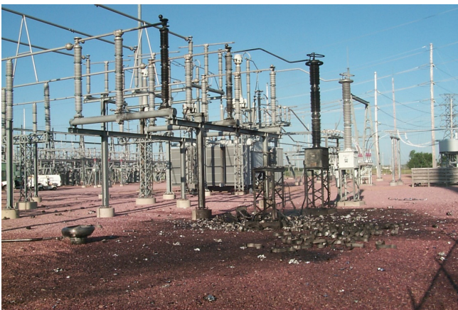
Fig. 38. Debris Scattered Throughout Substation Following a Catastrophic CVT Failure
