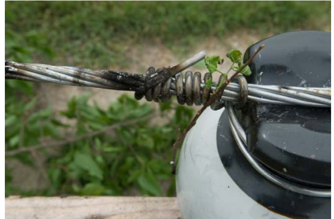
Fig. 11. Damage to Conductor, Experiment 3.
