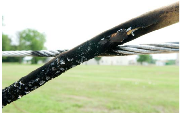
Fig. 3. Damage to branch and neutral conductor after Experiment 1.
