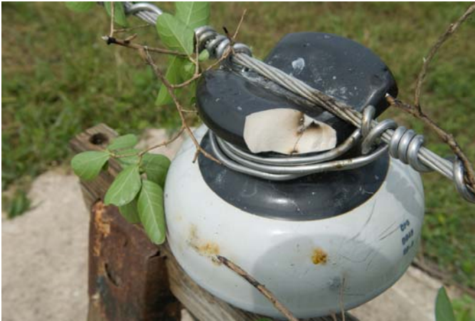
Fig. 5. Damage to insulator after Experiment 1.
