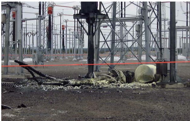
Figure 15: Picture of the remains of the CT
