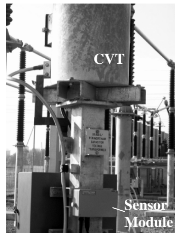
Fig 11.a- Sensor Module Mounted on a CVT Stand
