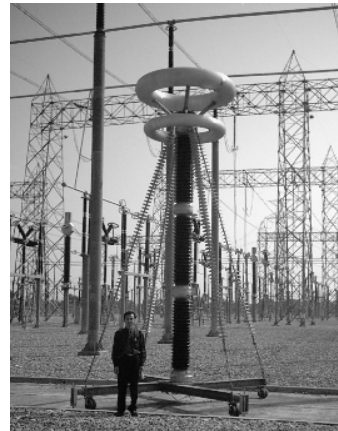
Fig 1- 500 kV Mobile Resistive Voltage Divider
