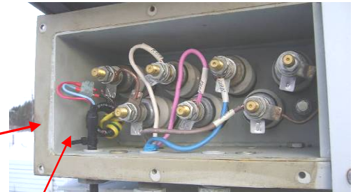
Marshalling box - Toroidal CT around the earth connection of the bottom capacitor
