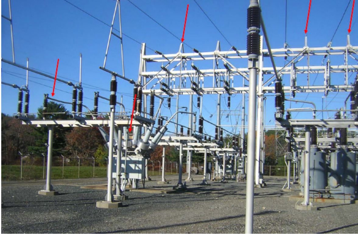
Figure 9 – I161 Line Bay (1612 CB foreground)
