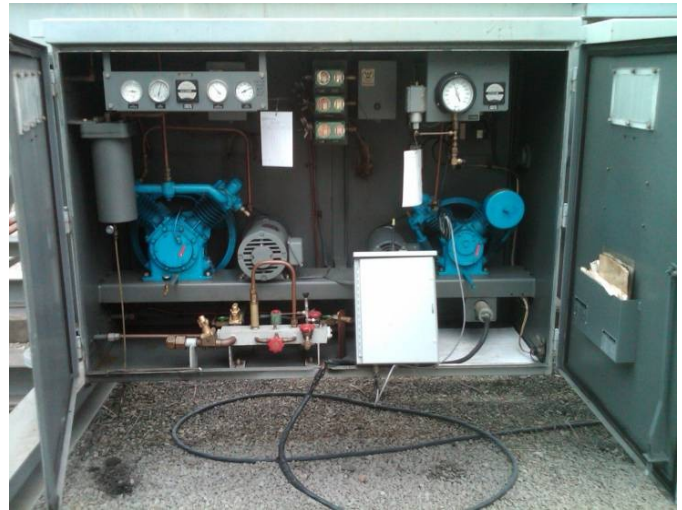
Fig. 7. The CBR device next to the open CB cabinet
