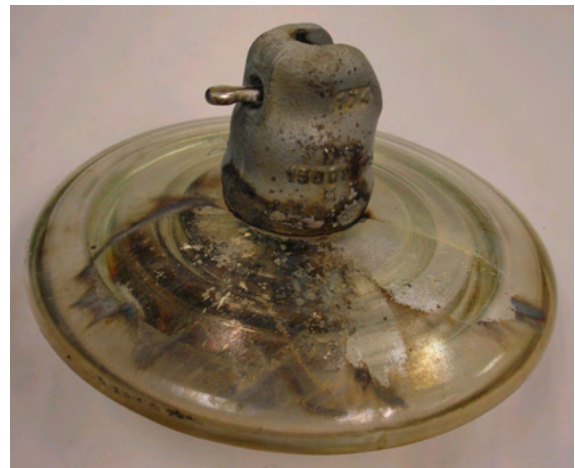
Fig. 29. Damaged insulator at 38.16 miles from the Goshen terminal.
