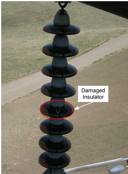
Fig. 26. Damaged insulator at 67.91 miles from Goshen terminal.
