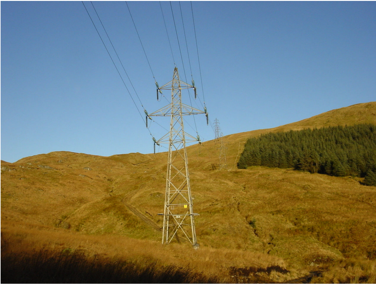
Fig 2 132KV Tower on the Dunoon Tee
