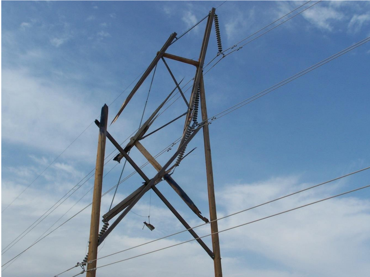
Fig 7 Structure Collapse Due to Fire Damage
