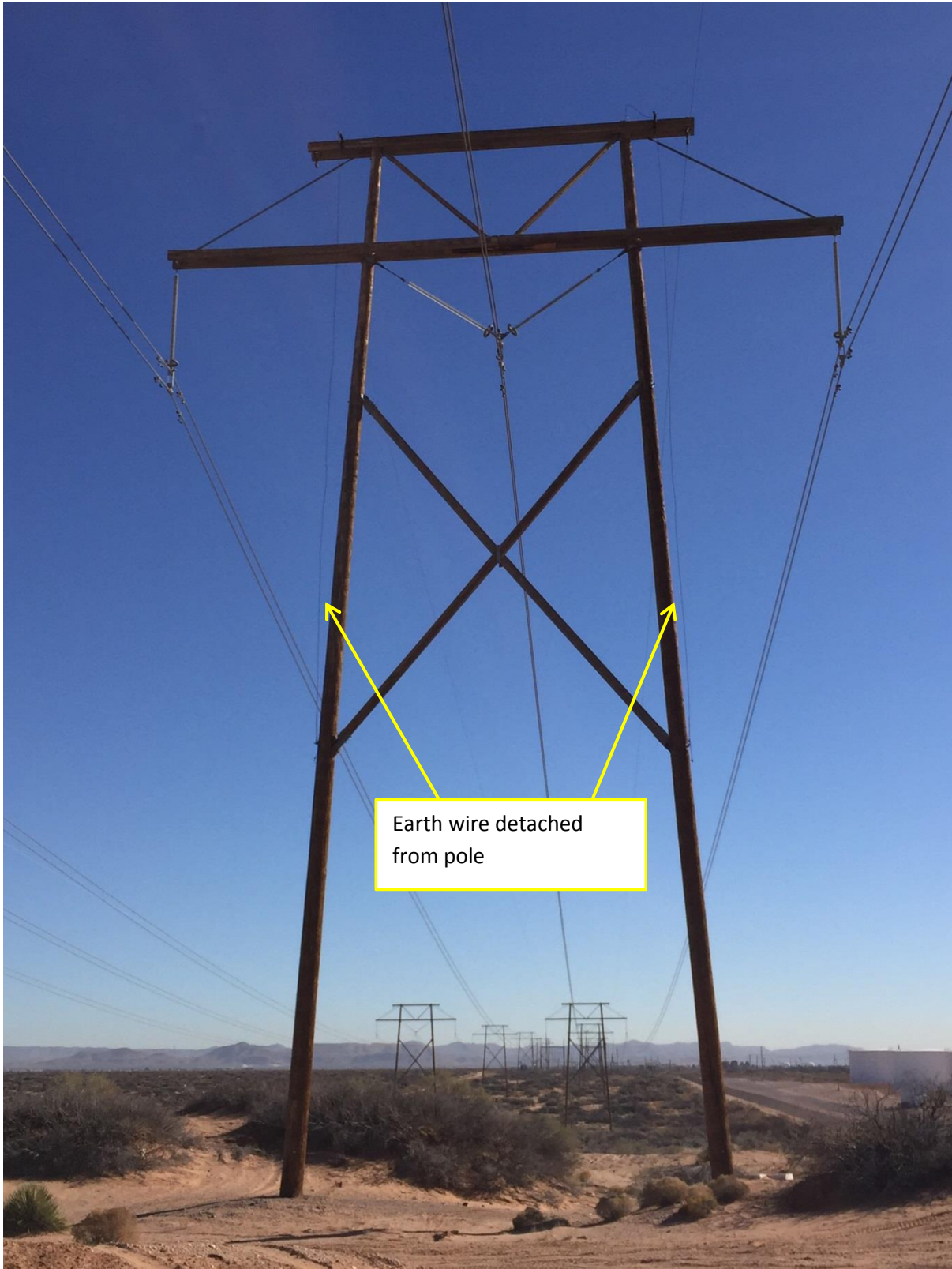
Figure 8 Design Upgrade on Earth Wire
