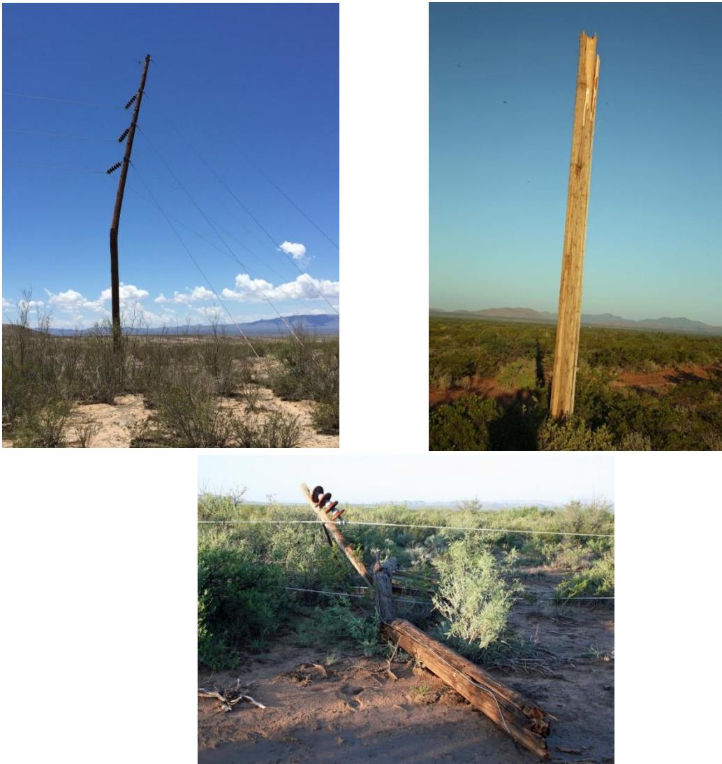
Figure 10 - 69KV Structures Damaged by High Wind Speeds
