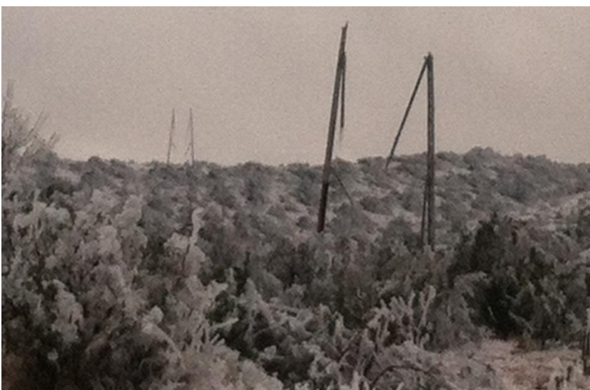
Figure 6 – Broken Structures due to Ice Storm
