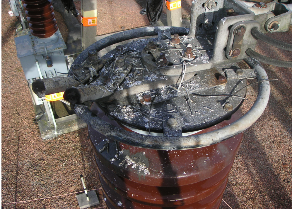
Fig 7 Top View of Failed VT
