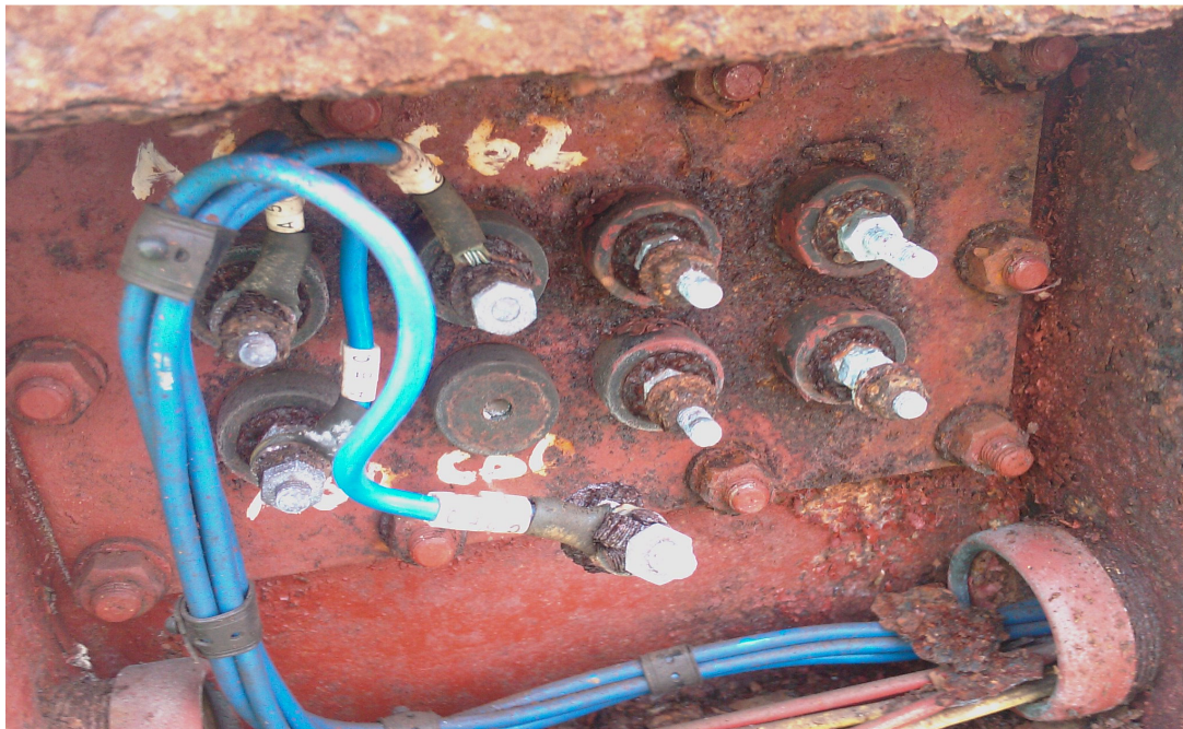
Fig 4 Badly Corroded CT Marshalling Box had an Intermittent Connection
