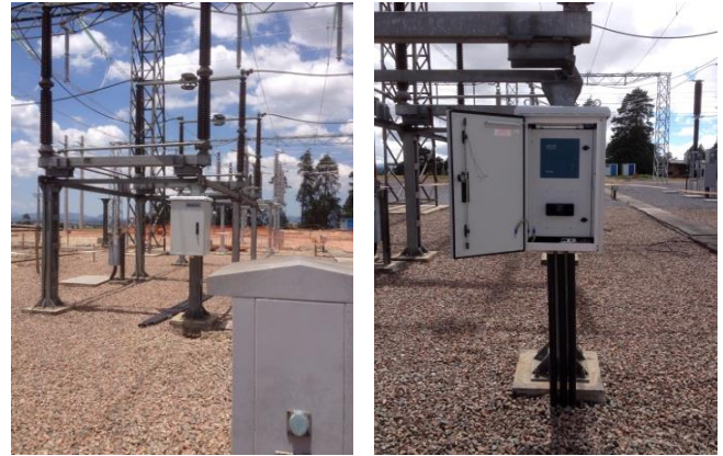
Figure 10: Field installation of MU320 panel at COPEL's Uberaba substation.
