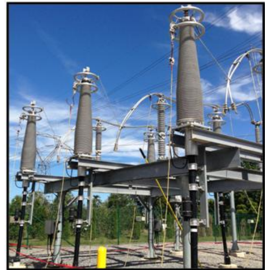
Figure 8 – Underground transmission line terminal where impedance measurements were taken.
