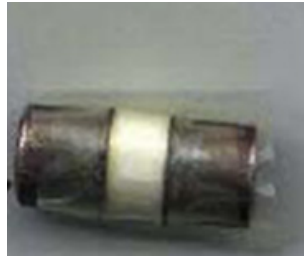
Figure 7 - Evidence of flash-over and heat damage
