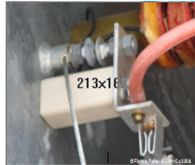
Figure 12 - More Flashover Mark
