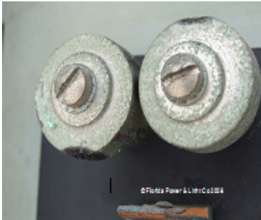
Figure 11 - Obvious Flashover Marks
