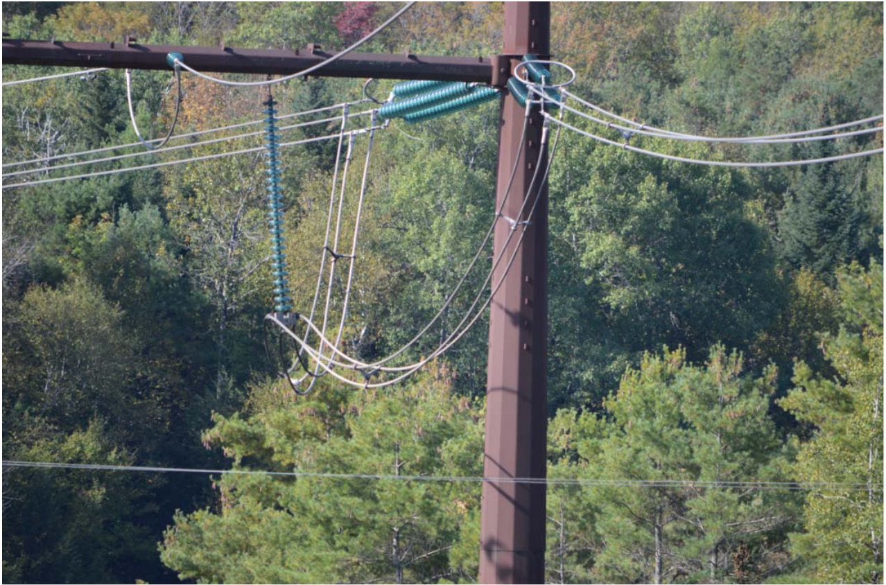
K60 Shield Wire Clearances
