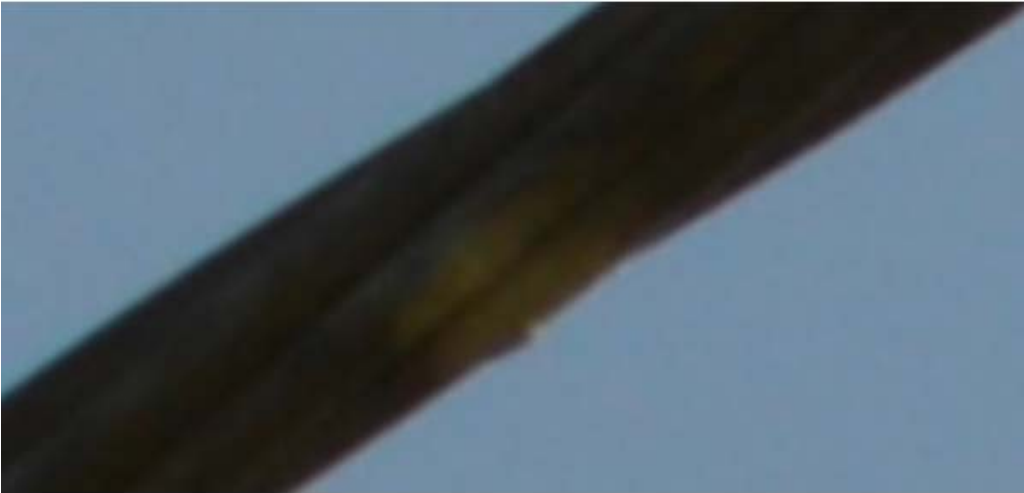
K60 Shield Wire Arc Mark
