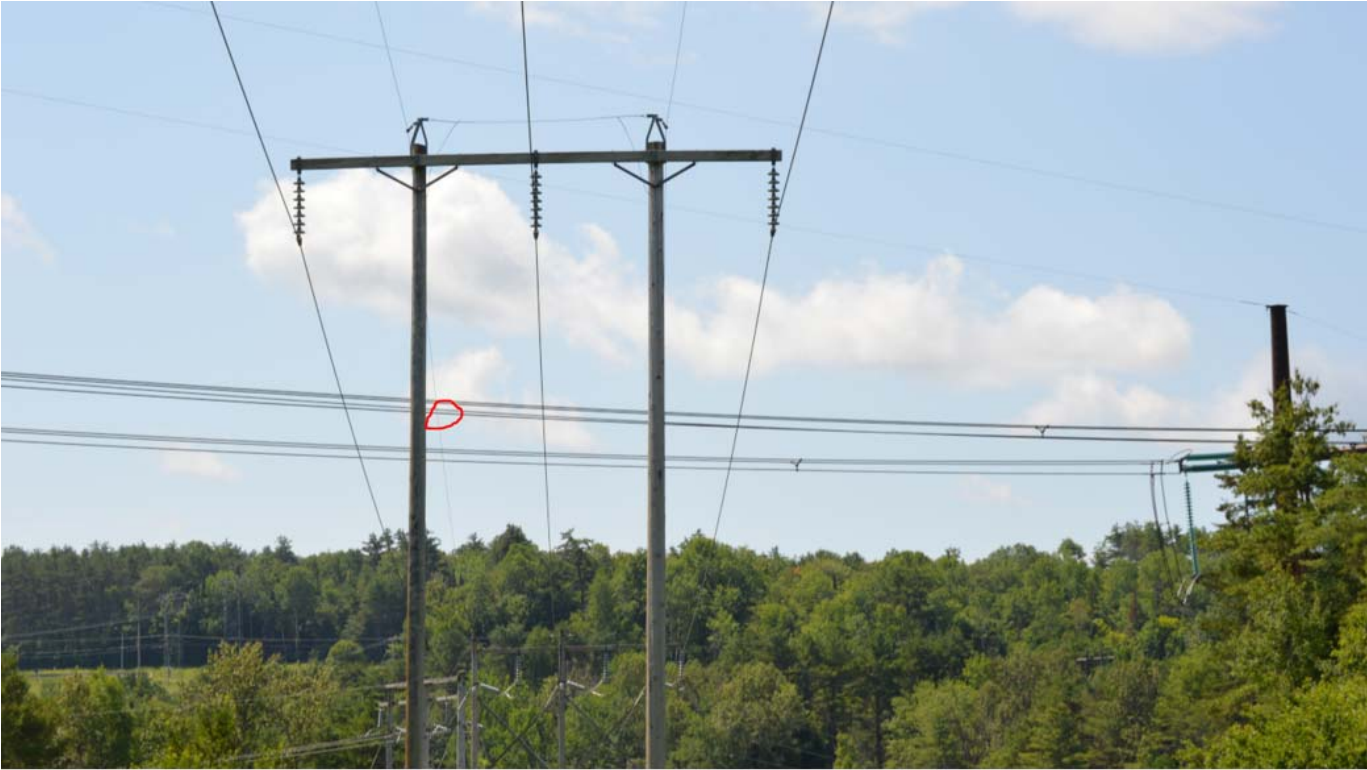
K60 – HVDC Line Crossing Fault Location
