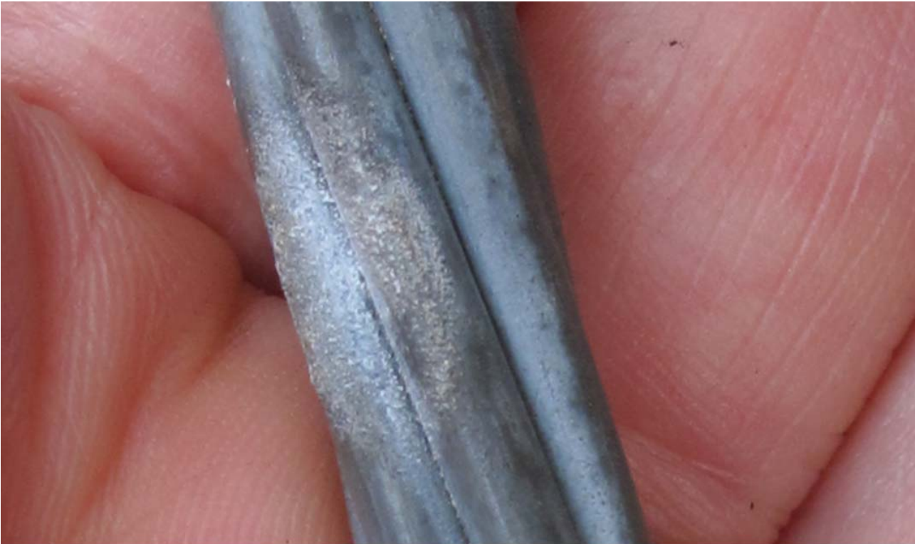
K60 Shield Wire Arc Mark #5
