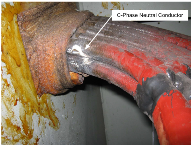
Fig. 29. Side view of the incoming and neutral conductors
