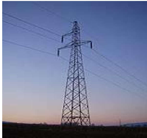
Figure 5 - Single Circuit Tower
