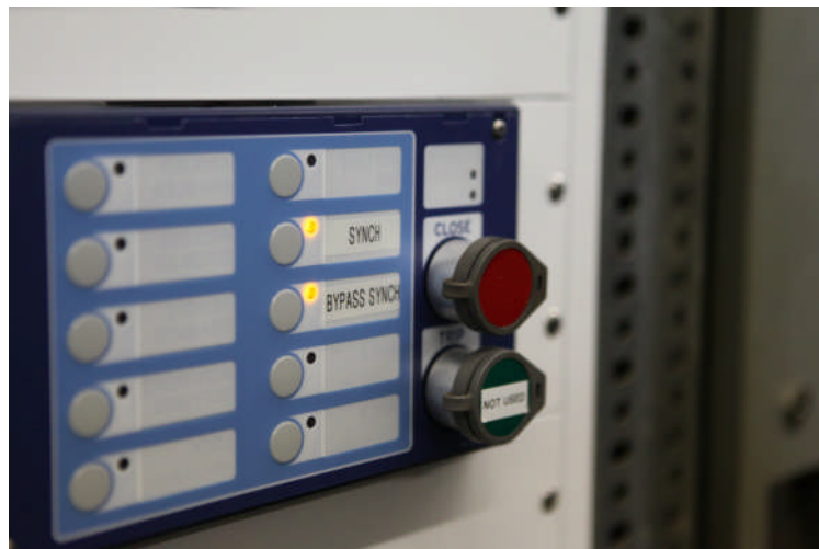
Figure 3: Microprocessor-Based Relay Used for Synchronizing
