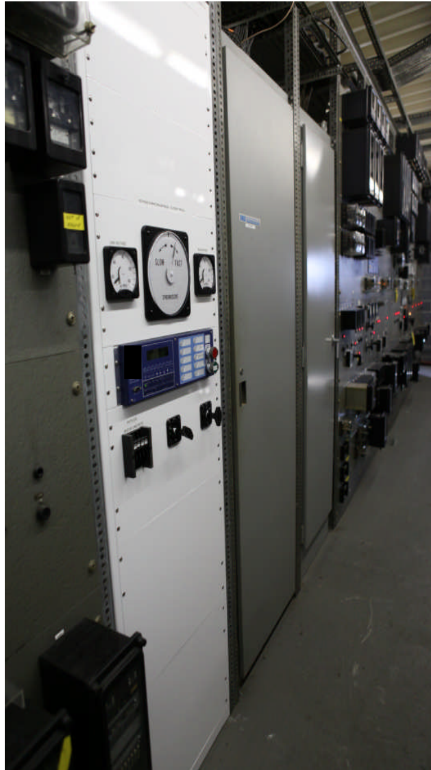
Figure 9: Synchronizing Panel Installed at the Substation
