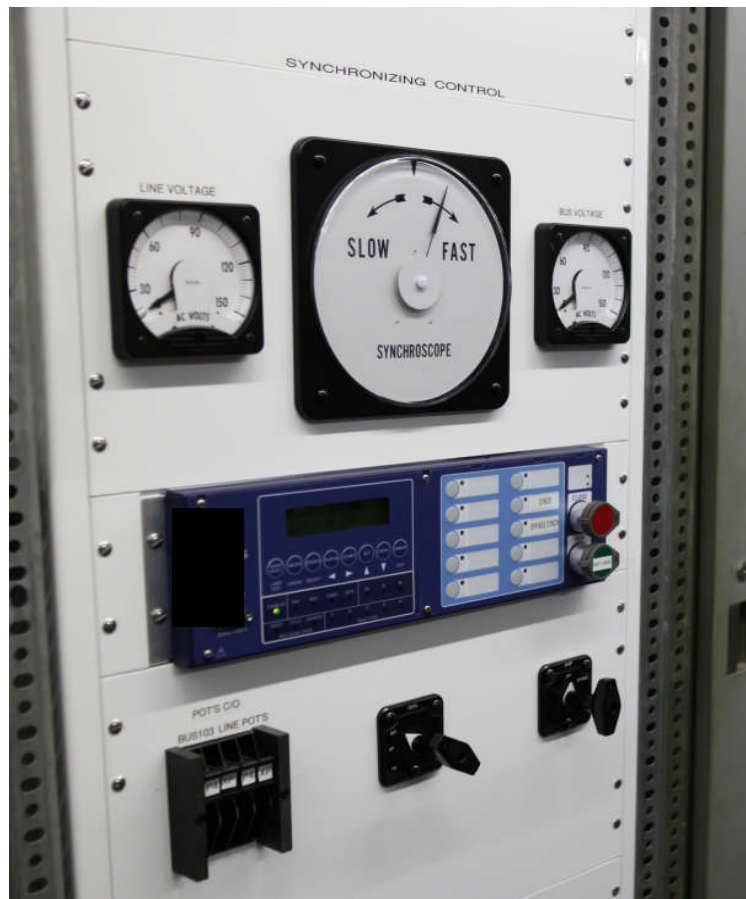
Figure 8: Close-Up of Panel Layout
