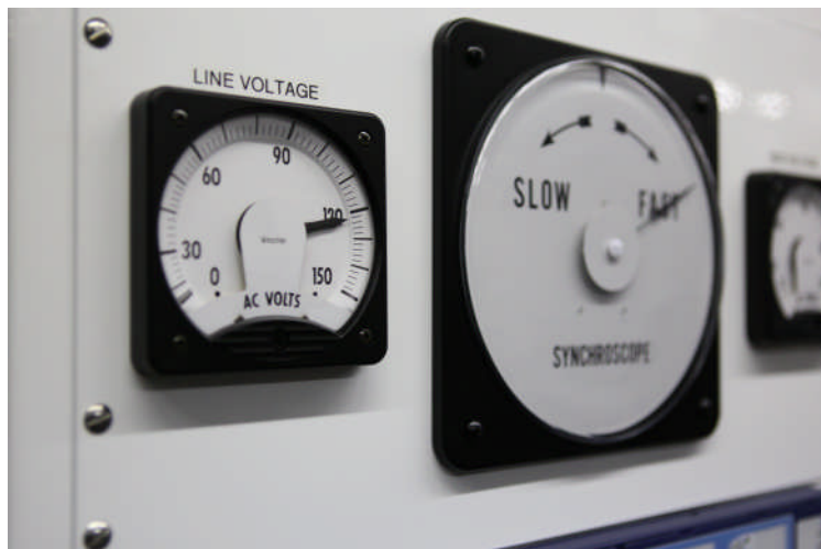
Figure 2: AC Voltmeter Measuring Line-Side Voltage Shown Next to the Synchroscope
