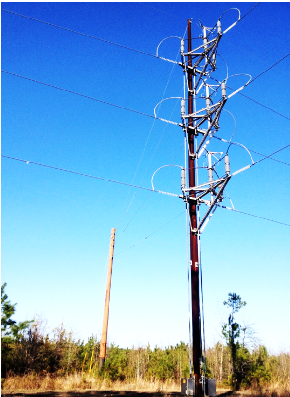
Fig. 2. Actual installation of ICS' and STU on a transmission line tap junction
