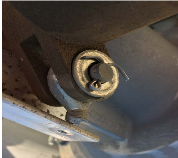
Figure 7 CB 212 rod-end eye bolt with retaining ring
