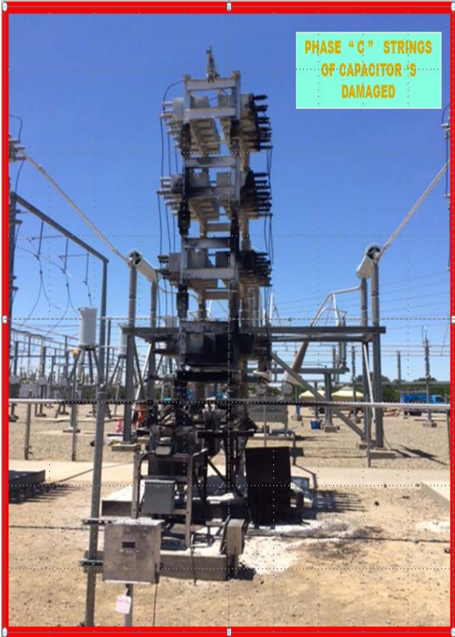
Figure 10 Capacitor Bank 1 with Phase "C" String Damage
