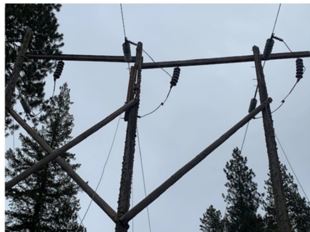
Fig. 9. Structure 32/3 temporary repair.
