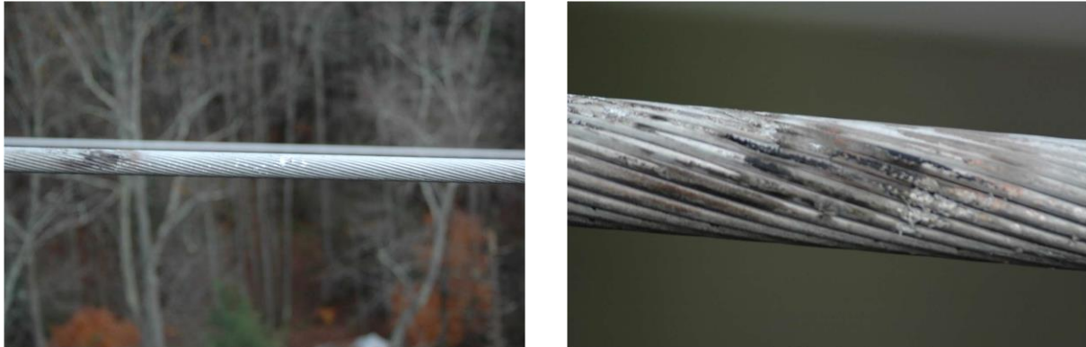
Figure 16 – Left - Mont-Susq conductor damage, Right – Close up of the conductor’s damaged strands
