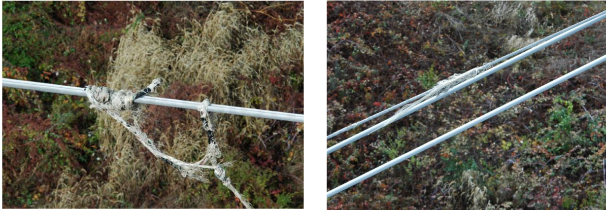
Figure 7 - Tether entangled on Sunb-Susq conductors, 500kV on left and 230kV on right
