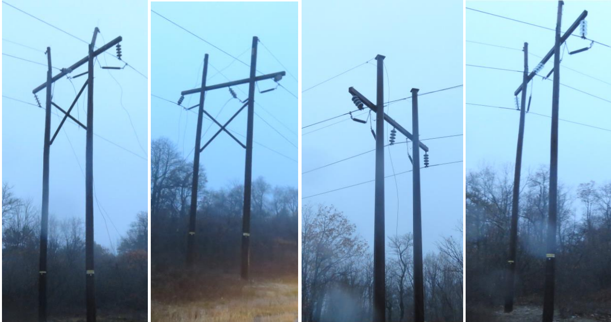
Figure 5 –Damages on Structures: 44894s55687, 44904s55715, 44868s55628, and 44879s55657
