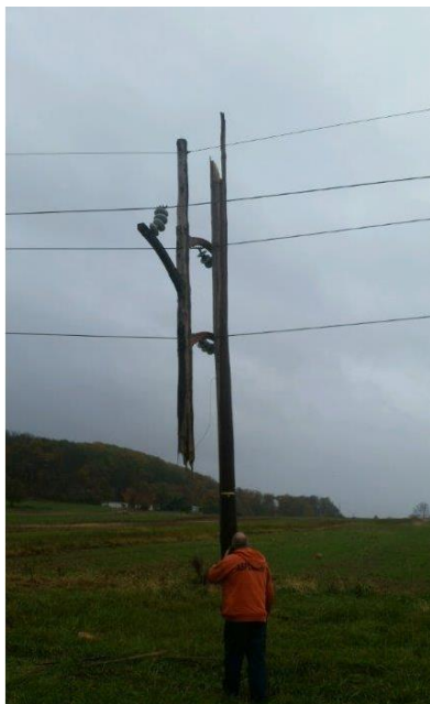
Figure 12 –Broken Pole on Colu-Scott
