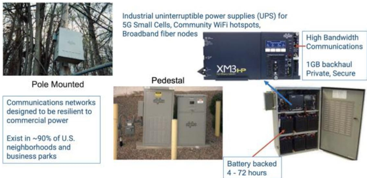
Figure 2: Broadband Network Industrial UPSs
