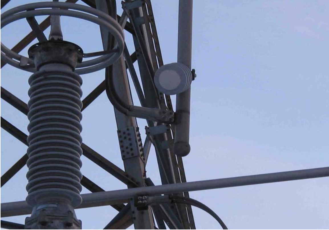
Picture 2: Broken Bottom Bus at Manchester
