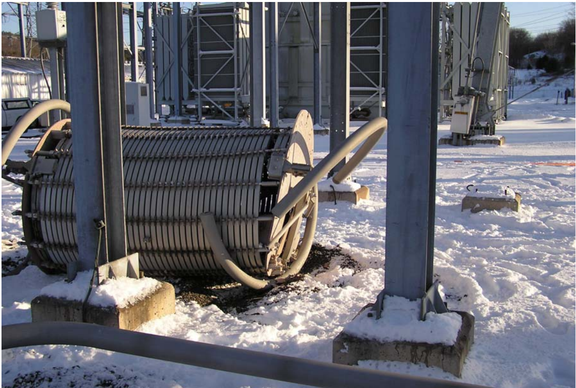
Picture 9: Fallen Trap at Frost Bridge
