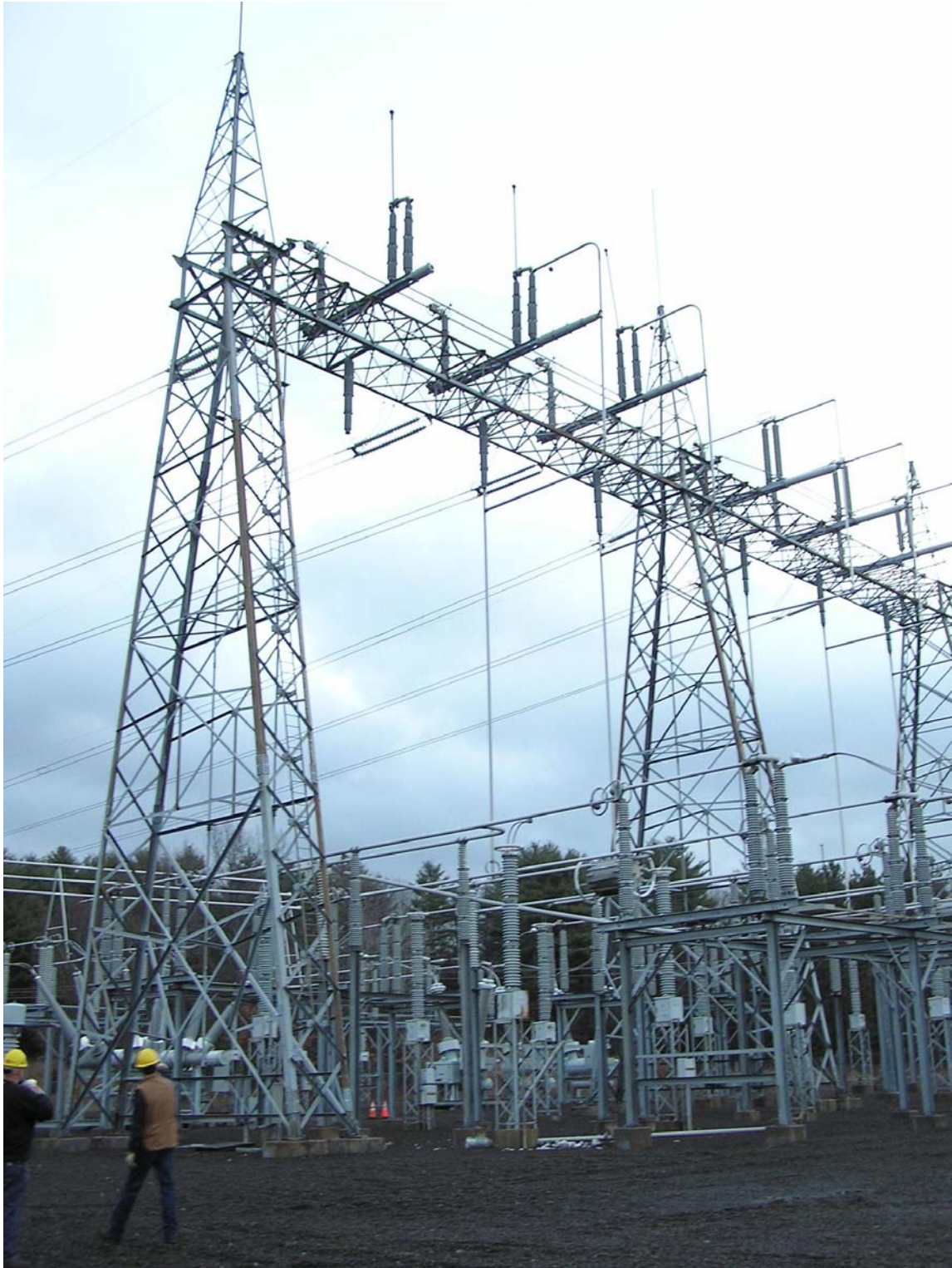
Picture 6: Missing Bus on Ludlow 334 Line Terminal
