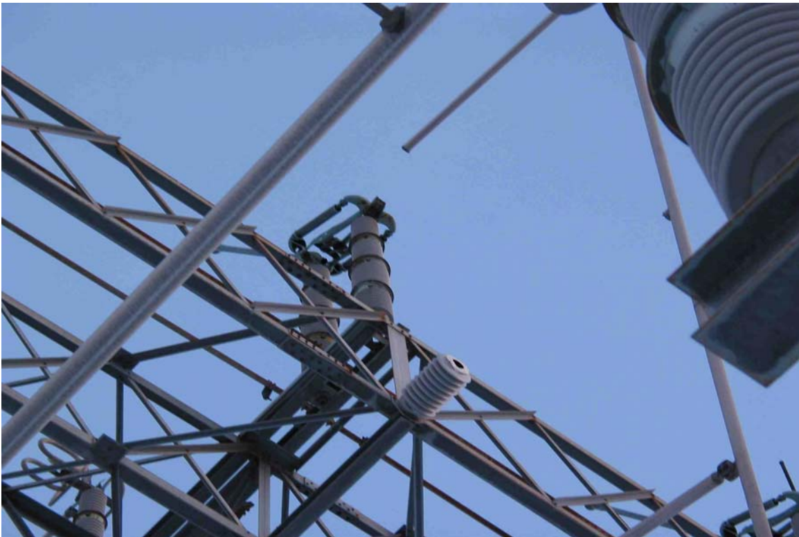
Picture 1: Open A Phase on Manchester 395 Line Terminal-Upper Bus End
