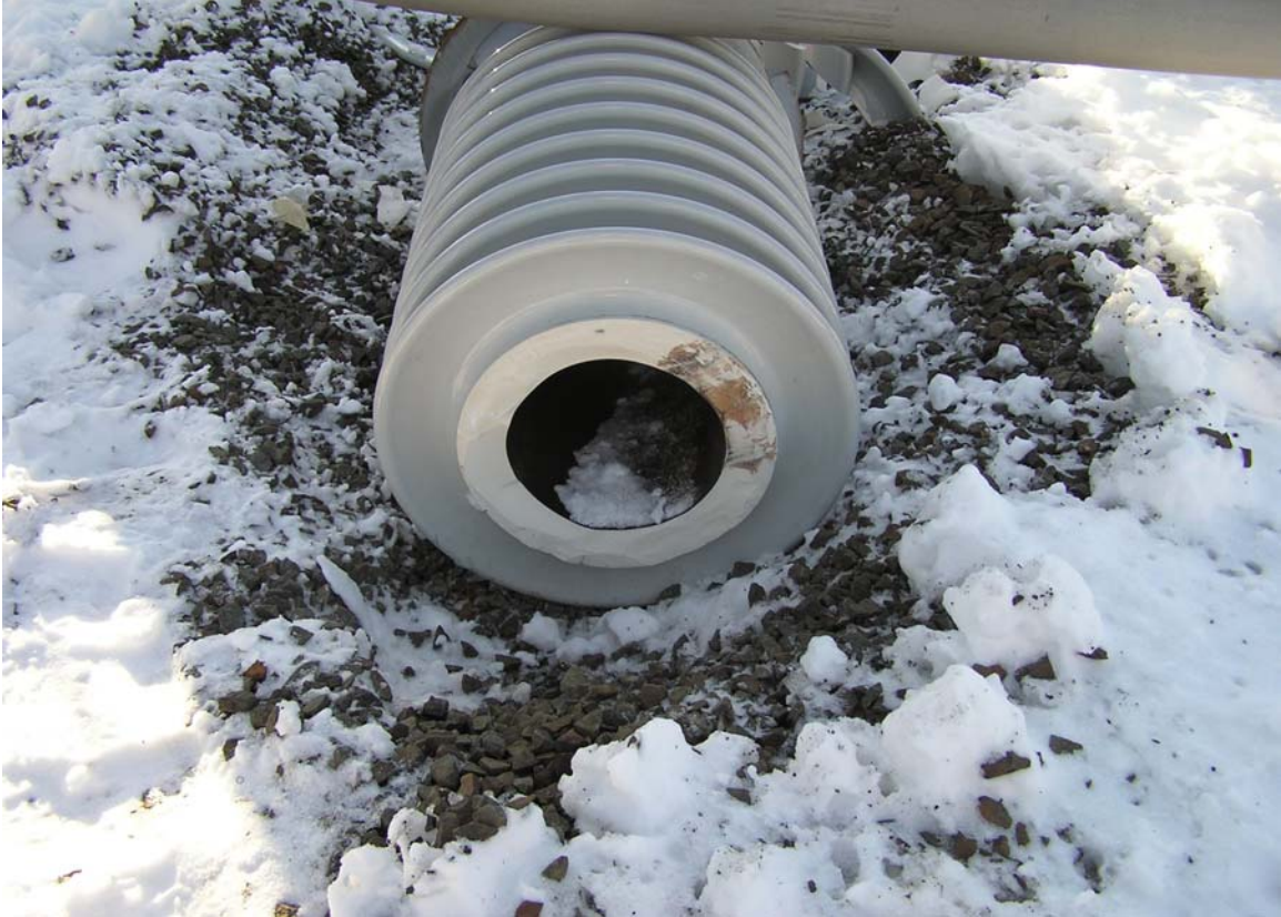
Picture 10: Failed Insulator at Frost Bridge
