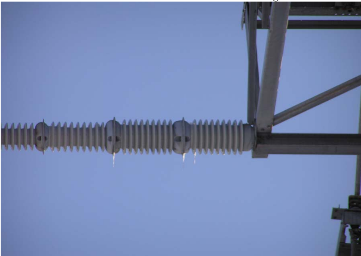
Picture 11: Ice Formation on Healthy Standoff Insulator
