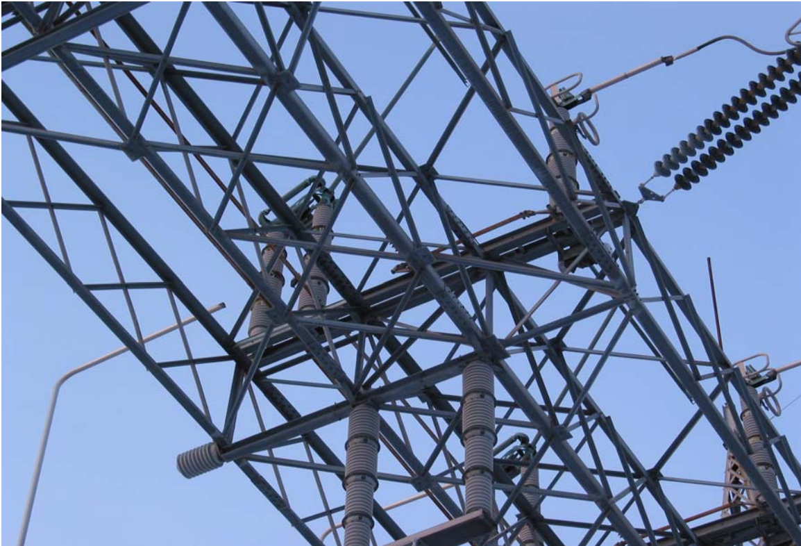
Picture 3: Another View of Open Phase A at Manchester
