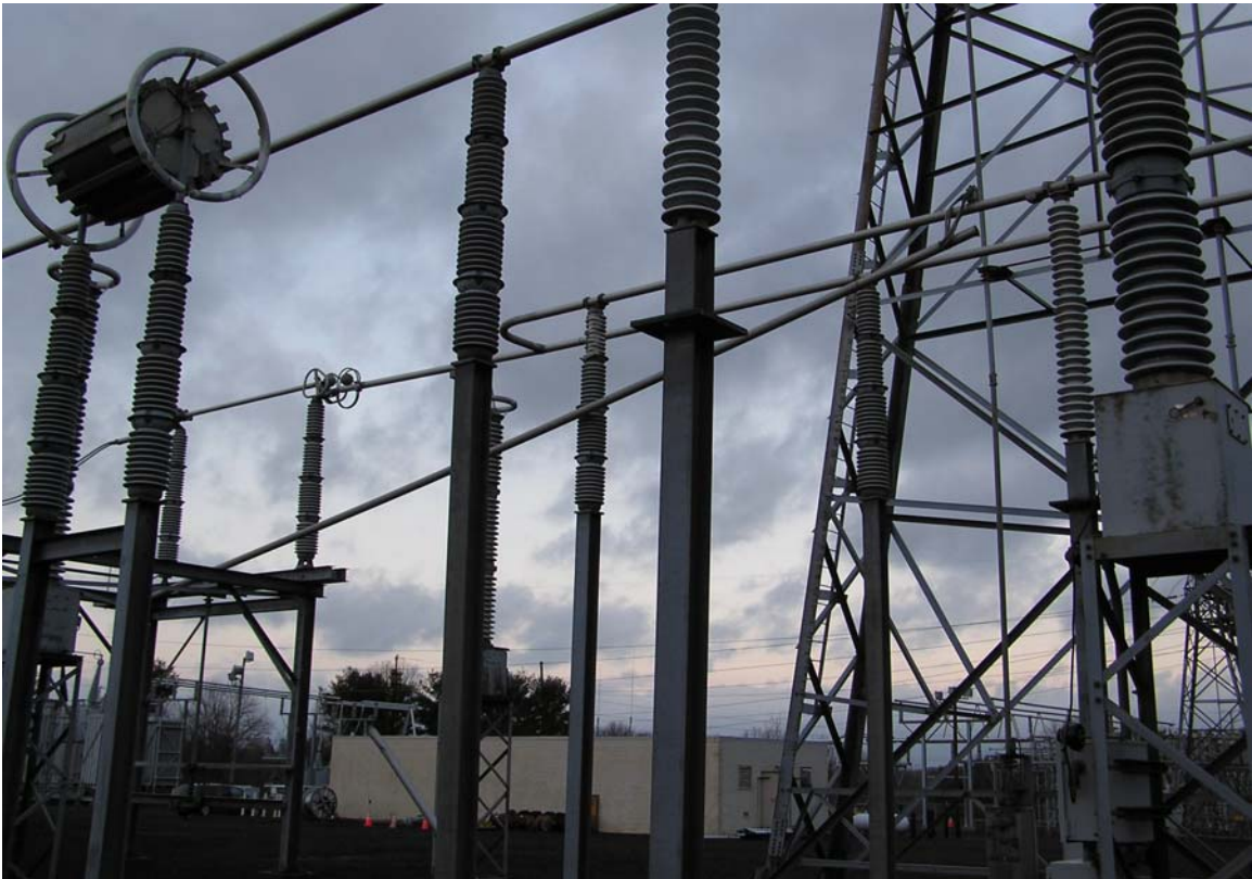
Picture 5: Ludlow 334 Line Bus Touching Live Parts and Ground
