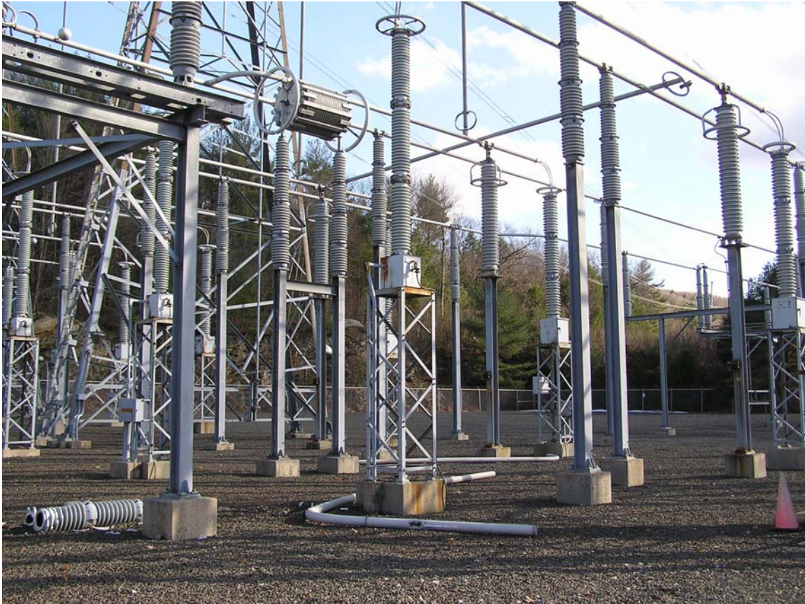
Picture 7: Northfield 312/393 Line Terminal Following Bus Insulator Failure
